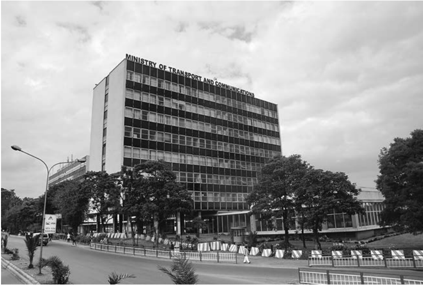
FIGURE 2.2. General Post Office and the Ministry of Transport and Telecommunications in Addis Ababa, codesigned by Štraus and Zdravko Kovačević in 1969. (Photograph by Brook Teklehaimanot Haileselassie, 2010)
