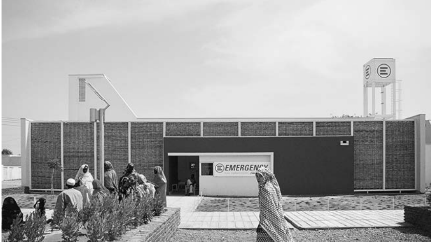
FIGURE 6.2. Pediatric Clinic, Nyala, Darfur, Sudan, 2010. Main façade with the shading system. (TAMassociati and Raul Pantaleo)
