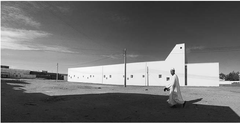
FIGURE 6.1. Pediatric Clinic, Nyala, Darfur, Sudan, 2010. Showing the south façade with small openings and the badger (the chimney-like structure on the right side of the building). (TAMassociati and Raul Pantaleo)
