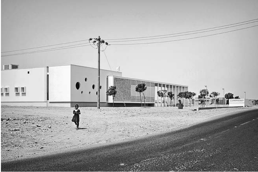
FIGURE 6.3. Pediatric Clinic, Port Sudan, Sudan, 2012. The clinic in its dusty context. On the right are the locally sourced natural-fiber shading panels that form part of the building envelope. (TAMassociati and Massimo Grimaldi)
